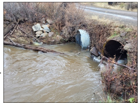
Above, two aging, inadequate culverts contributed to flood risk and erosion in Thorn Creek. Below, the new squash culvert will better accommodate high flows and minimize erosion.
