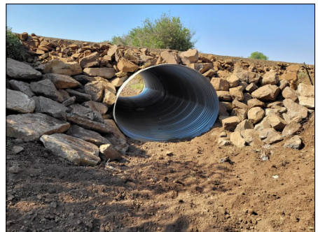
Above, two aging, inadequate culverts contributed to flood risk and erosion in Thorn Creek. Below, the new squash culvert will better accommodate high flows and minimize erosion.
